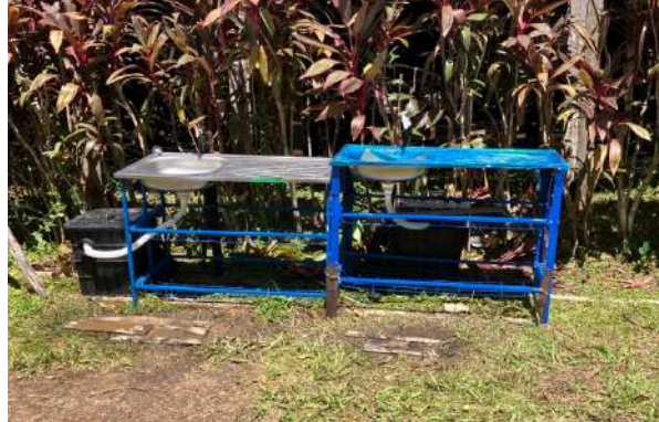
Photos 7 & 8: Grease trap placement and installation near vendor's kitchens and food stall areas
