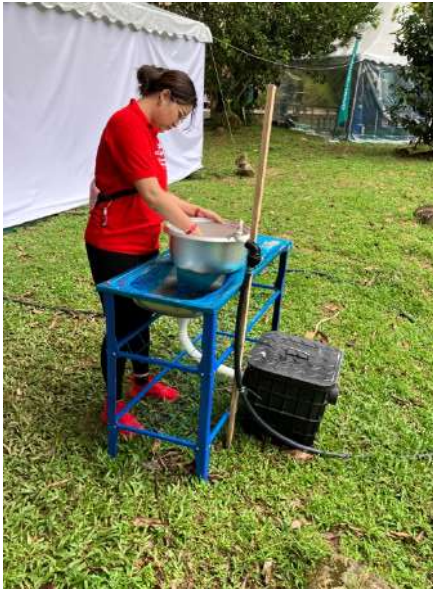
Photos 7 & 8: Grease trap placement and installation near vendor's kitchens and food stall areas
